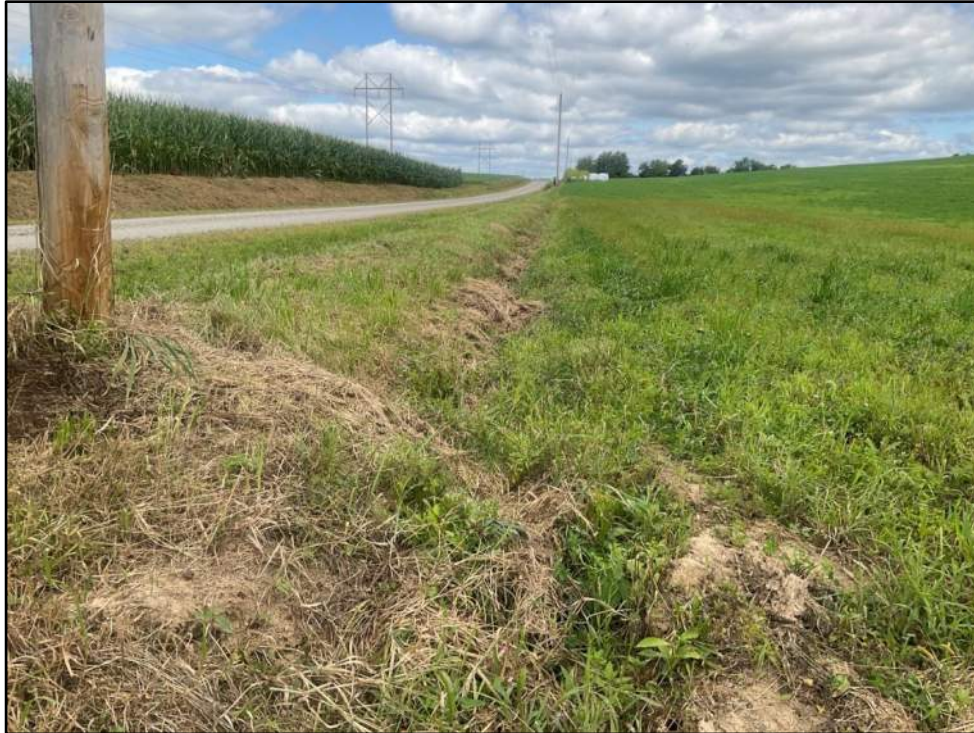
Photograph 1. Stormwater Erosion, SWE-AGS-004 (Ditch), Facing North
